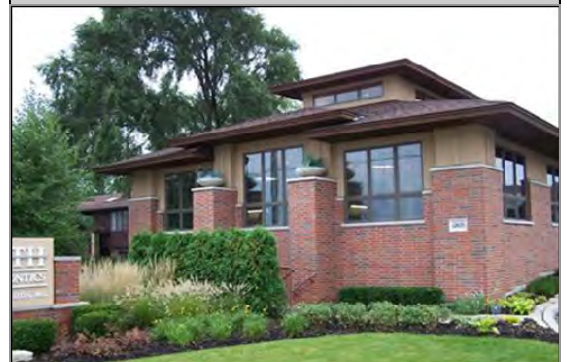
Masonry is carried up the vertical, heavy columns to emphasize their size and provide an accent on the façade. The color of the bricks provides a range of tones, which creates depth and texture on the façade.
