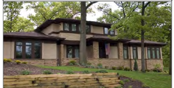
The contrasting colors, materials and textures create a distinct base, middle and cap with transition details between each layer.
