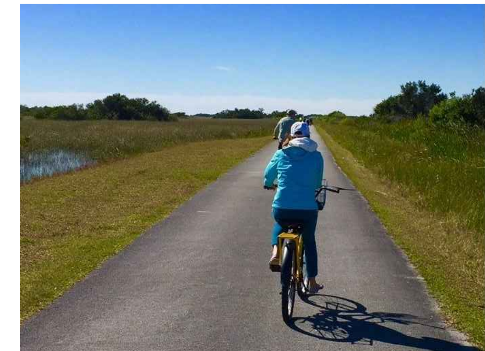
ASPHALT BIKE PATH
